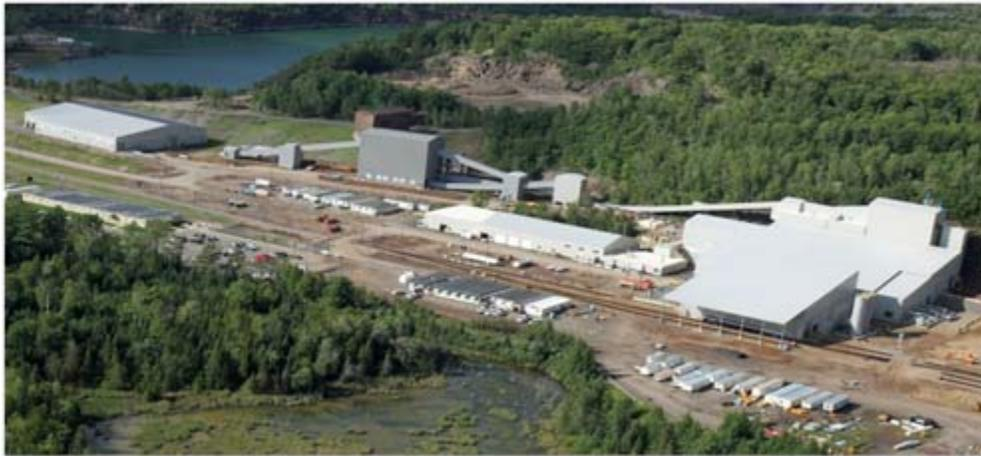
Lundin Mining chose to install a *WirelessHART* network to monitor and protect its essential equipment. The flexible, yet robust wireless system addressed critical applications ranging from freeze protection for fire systems, to monitoring the health and performance of sump pumps and crushing equipment. The use of wireless technology also helped the mill substantially reduce installation costs and avoid failures.
