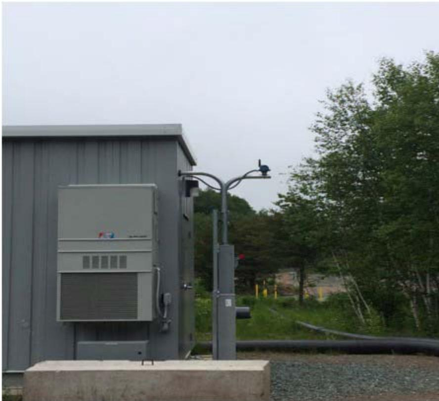
Since its installation in late 2014, the *WirelessHART* network has provided for reduced start-up times along with the assurance that all is well in the mill's remote locations. The
