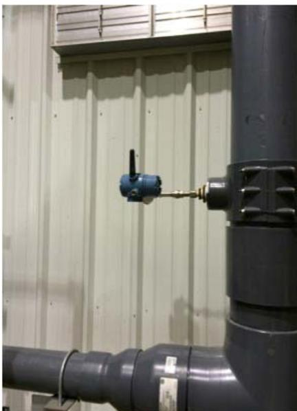
The AMS Device Manager was networked with Emerson's Machinery Health Manager software to provide a comprehensive monitoring and management tool for smart devices, including wireless vibration transmitters used to monitor the condition of crushers and ball mills. This solution improves reliability and supports preventative maintenance programs. Vibration analysis data can be pulled from history each day, and alarms are generated from the vibration equipment.
