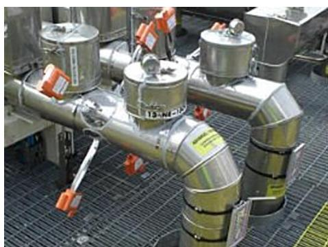
Today, researchers can opt for permanently installed, wireless ultrasonic wall-thickness-monitoring sensors for corrosion monitoring. The units generate, on a continuous basis, the data required to make proper decisions and provide this information directly to plant personnel.
