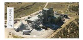
Natural Soda recovers sodium bicarbonate using a process known as solution mining. This involves pumping heated water 1,900 feet underground to dissolve nahcolite beds and form a brine solution that is pumped to the surface and sent to the production plant.
