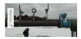
The most important result of using *Wireless*HART flow, pressure, and temperature transmitters at the well pads is that operators can confidently deliver expected production results with no leakage into the freshwater aquifer. The system works flawlessly to protect the environment.
